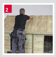
If you are replacing the roof, check that the existing felt is not unduly wrinkled, smooth out any bumps.
