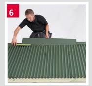
Place the ridge pieces on the top of the roof and overlap to ensure they extend from one end to the other, if necessary covering any existing timber barge boards.
