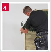
Nail through the top of the corrugation into the existing boarding using the nails provided.
