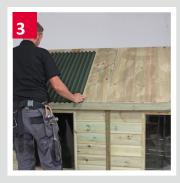
Start by placing one of the sheets to the left hand side of the building, allowing no more than a 20mm overhang.
