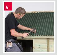
Place the next piece to the first with a two corrugation lap and fix as before.
